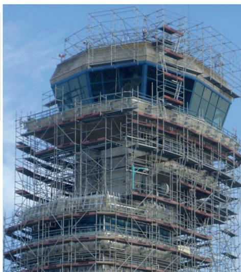
FLEXIBILITÉ ET ADAPTABILITÉ AUX DIFFÉRENTES CONFIGURATIONS DES BÂTIMENTS GRÂCE AU SYSTÈME DE "ROSACES"
